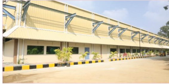
PROJECT Turnkey Project YEAR OF COMPLETION 2022 LOCATION Nuclear Fuel Complex, Hyderabad SPECIAL FEATURE 40m clear span structure with 4 cranes, walk way, with extension and linking with existing shed. Project with complete civil work, infrastructure, Fire Fighting and PEB Structure
