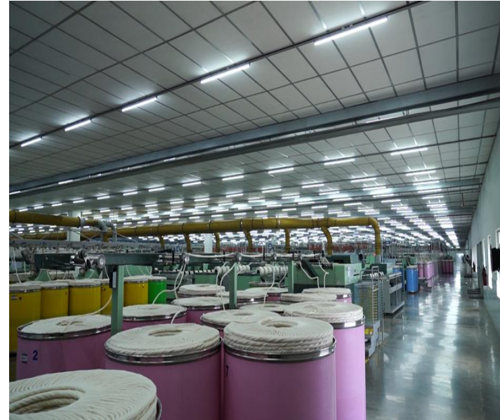
Electrification work of Spinning Mills
