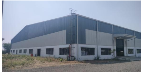
PROJECT Industrial Shed YEAR OF COMPLETION 2024 LOCATION CH.SAMBHAJINAGAR SPECIAL FEATURE - Multi Span Industrial Shed Of 80, 000 Sq.Ft at Ch.Sambhajinagar
