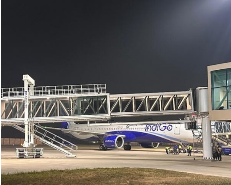
Passenger Boarding Bridge
