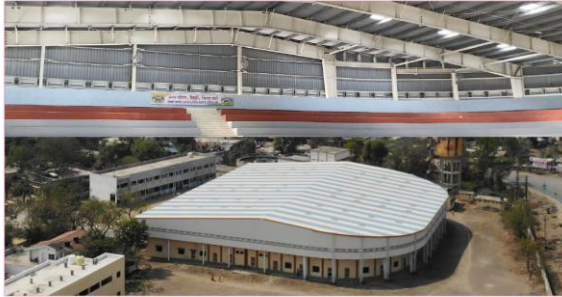
PROJECT Indoor Stadium YEAR OF COMPLETION 2016 LOCATION Deoli, Wardha SPECIAL FEATURE Clear Span Structure of 62m, with complete civil works and seating capacity of 3,000 peoples.
