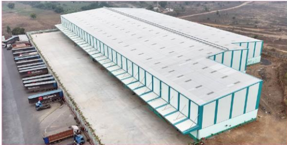
PROJECT Logistic Warehouse YEAR OF COMPLETION 2023 LOCATION Kalameshwar, Nagpur SPECIAL FEATURE 150,000 Sq. Ft. Warehouse with 12 m. clear height & continues ridge-vent & insulation
